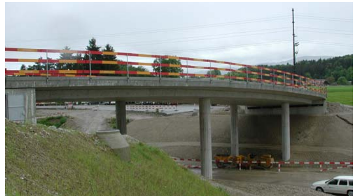
Figure 1. View of the bridge.
