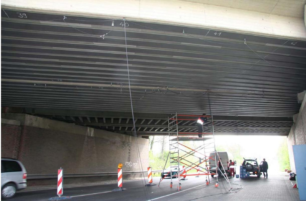
Figure 9. View underneath the Erfttal Bridge on measurement day 1. From left: Traffic lane open to traffic, closed traffic lane, paved “green strip” where the black measurement van is located, bicycle/pedestrian lanes.
