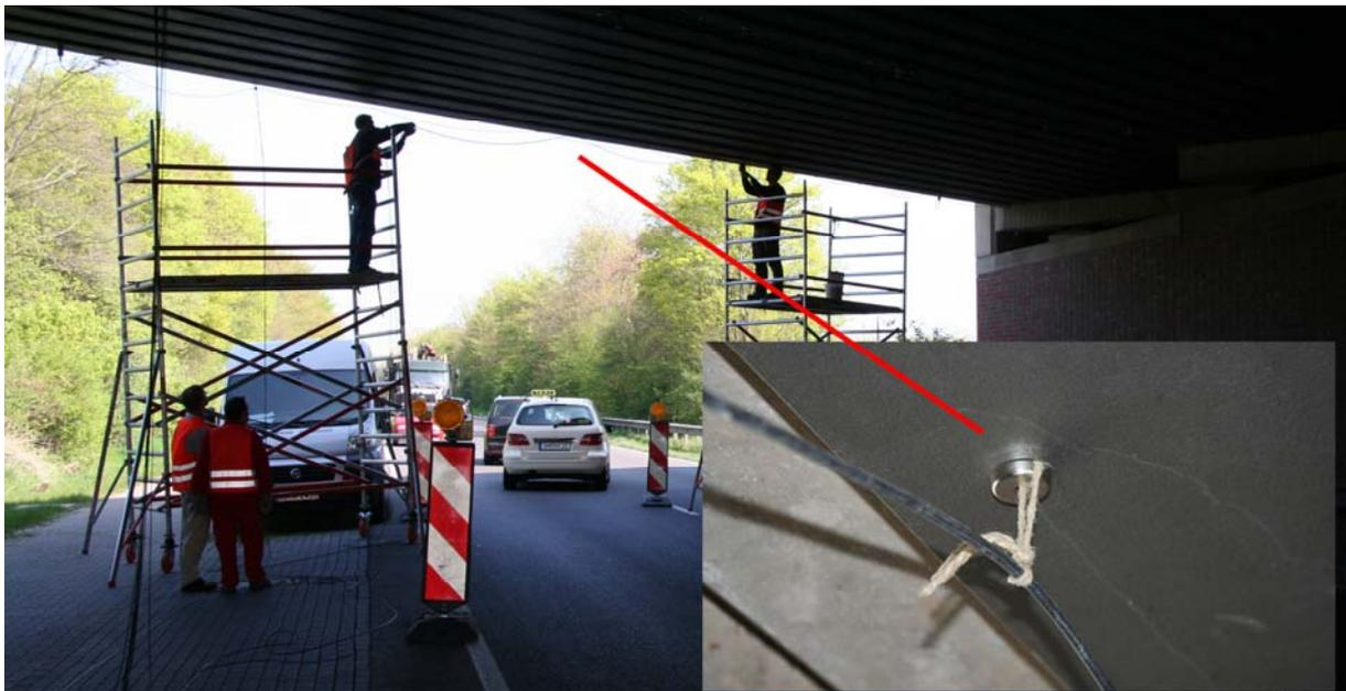
Figure 10. View underneath the Erfttal Bridge on measurement day 2. View direction reverse to the one in Figure 9. The detail in the right hand corner illustrates the technology used to fix a “flying” cable to a steel beam.
