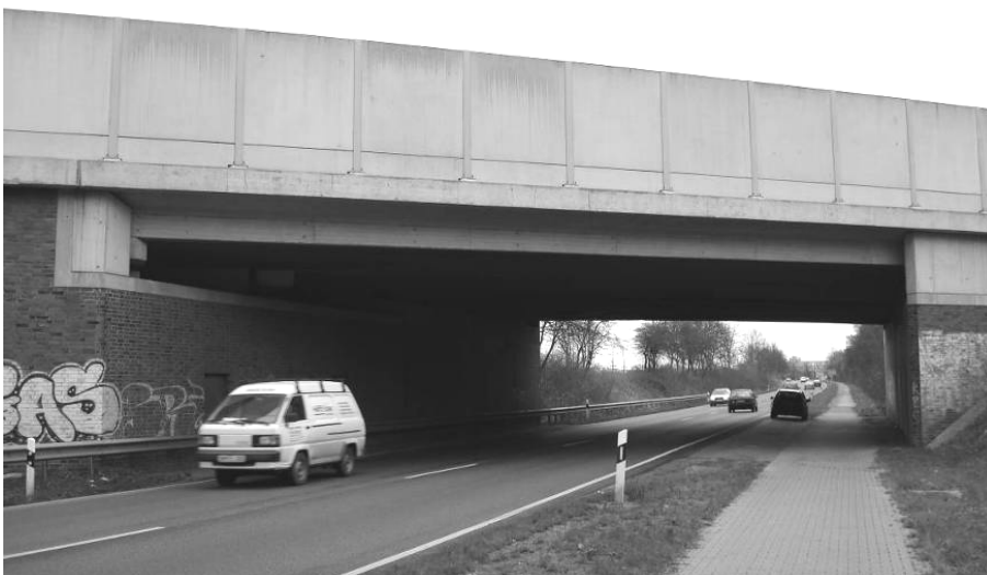
Figure 1: View on the filler beam bridge “Erfthal Bridge” near Kerpen, Germany
